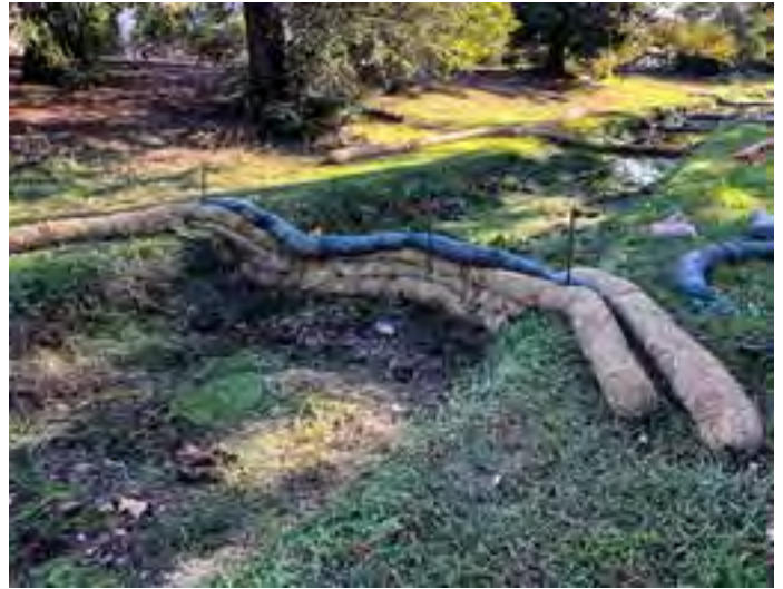
The green wattle atop this water barrier has been inoculated with mycelium, the weblike network of fungi that sprouts mushrooms. The wattles reduce the flow on the creek, allowing for less turbidity and longer uptake of toxins.
