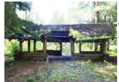
View of current Crystal Springs Forest Camp CCC shelter looking south. The large central opening is where the stone fireplace and chimney used to be.
