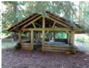
Side view of current shelter looking east.
